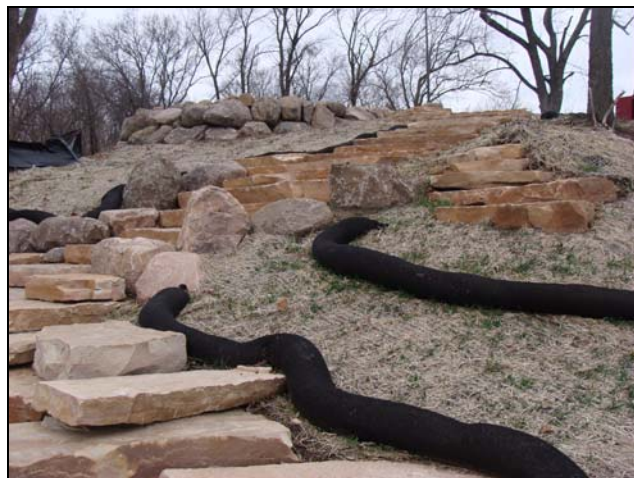
New Picnic Point Stairway to Lake Mendota, 2012 (R James)
